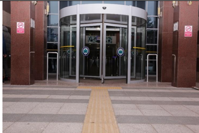
There is a relief path from the outside to the entrance of the library. (Eskişehir Osmangazi University, Türkiye)
