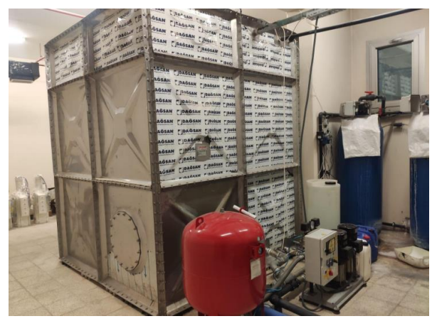
Groundwater well pumps and storage
